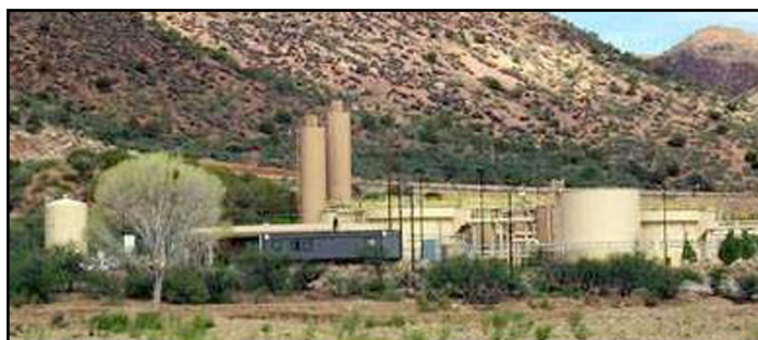
Lower Pinal Creek Treatment Plant.
